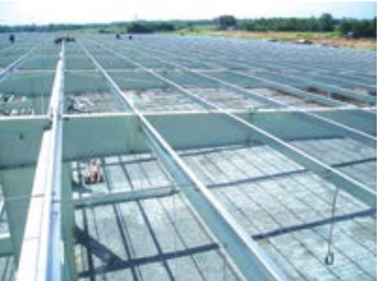
SECONDARY MEMBERS (Minium Yield Strength is 34.0 kN/cm 2 )
