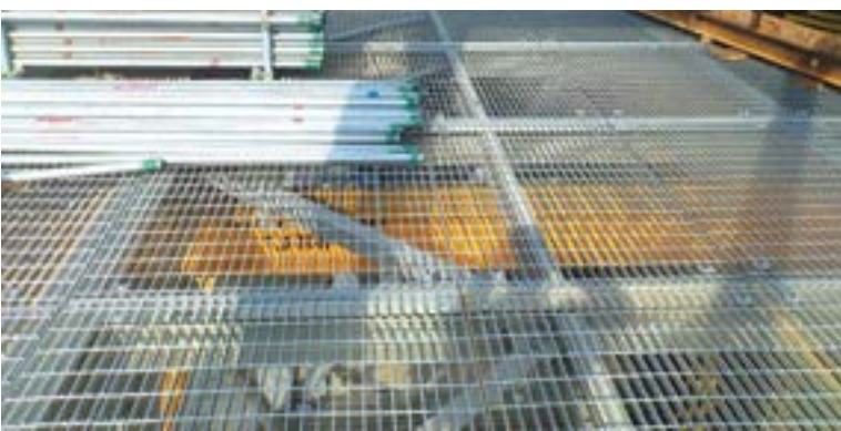
MEZZANINE GRATING CONNECTION TO JOIST
